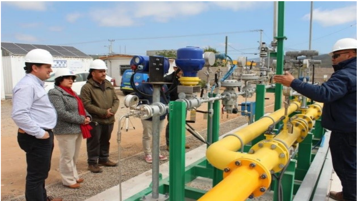
Inspection of the pilot plant H2GN of Gas Valpo. Coquimbo, December 2023
